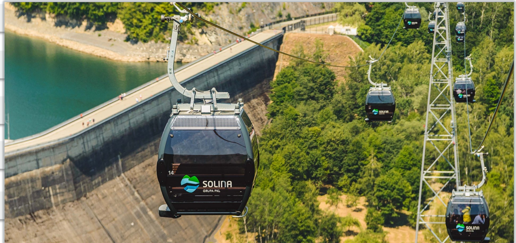
Solina dam cablecar (Source: PKL)
